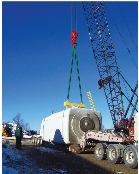
Wind Turbine Installation
