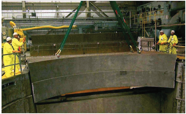
Nuclear Reactor Containment Sections
