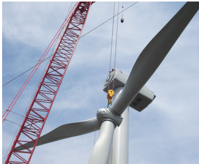
Wind Farm Construction
