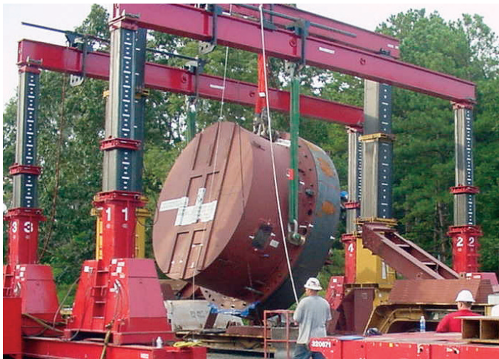
Nuclear Reactor Head Turning
