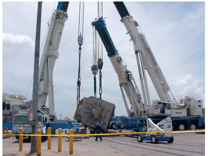
Electric Generator Recovery
