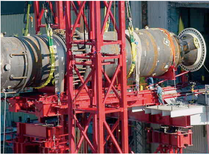
500 ton Steam Generator Replacement
