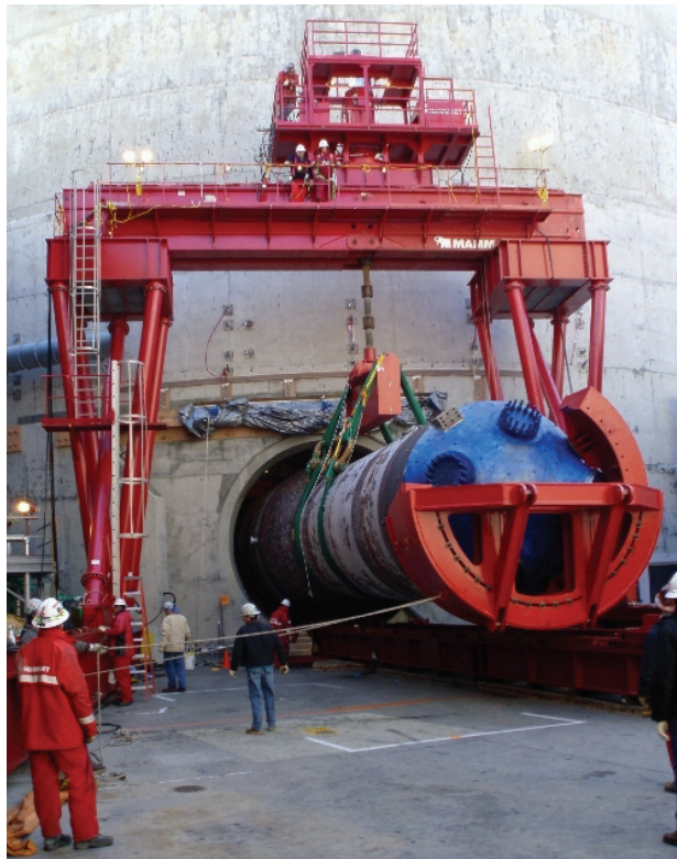
Steam Generator Installation
