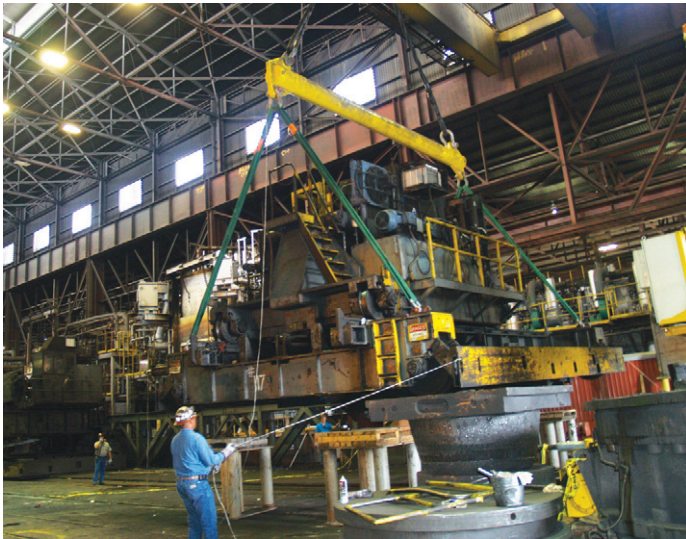
Steel Forging Plant Maintenance
