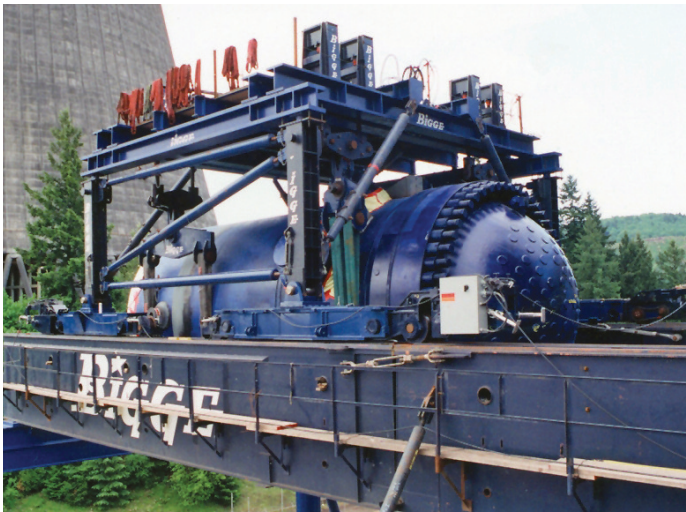
Nuclear Reactor Removal
