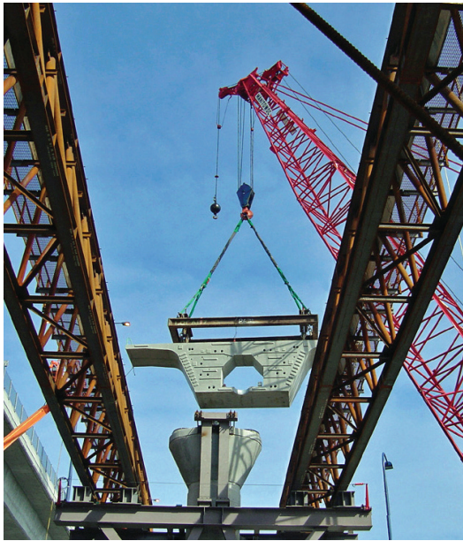
100 ton Bridge Section
