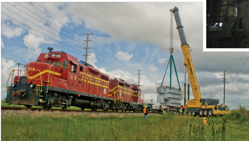
Power Transformer Installation
