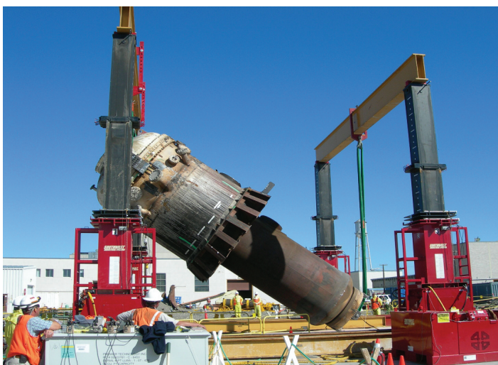
Test Reactor Removal
